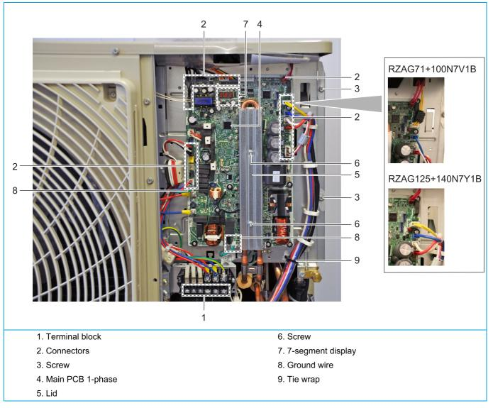
Secondly, strip the Main PCB assembly (front)
