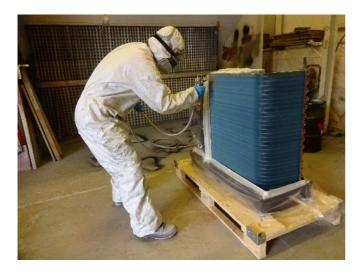
Blygold PoluAl is an anti-corrosion treatment consisting of a conversion layer followed by a polyurethane top coat. The operating temperature range is from -20°c to 150°c. The Blygold treatment can be applied to cooling and DX coils.
