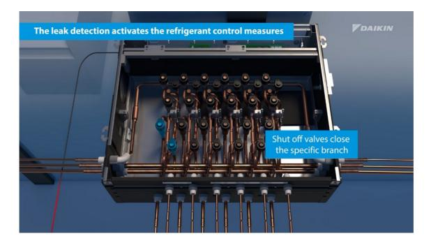
Automatic, real-time refrigerant leak detection and containment controls are another outstanding feature of the new VRV 5 thanks to built-in Shîrudo Technology which is designed to ensure that any potential refrigerant leak is quickly detected and isolated – greatly reducing direct emissions impact.
