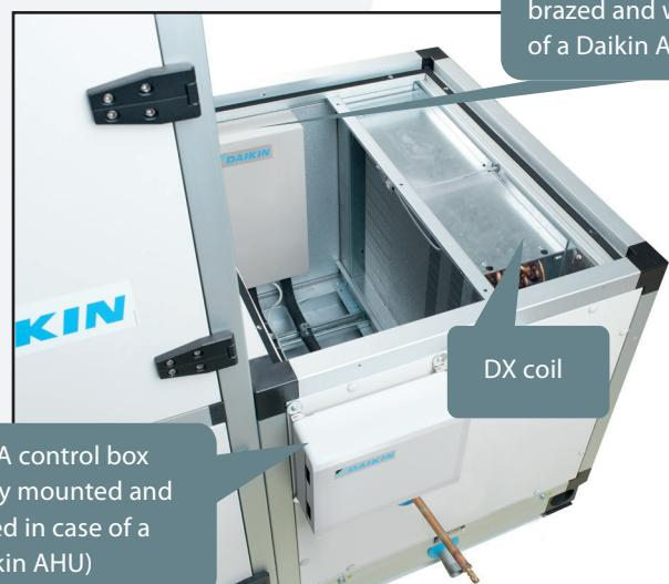
**EKEXVA** electronic expansion valve (fully brazed and wired in case of a Daikin AHU)
